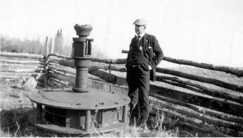
*2008.008/19—WB in 1928, posing beside the water turbine pulled up on shore.*
